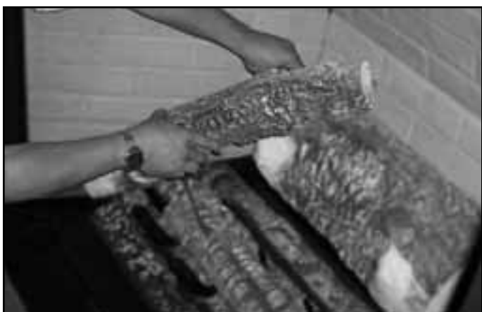
Figure 14.13 Positioning Left Log
